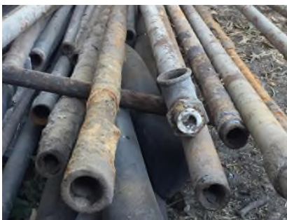
Old water pipes showing blockage
