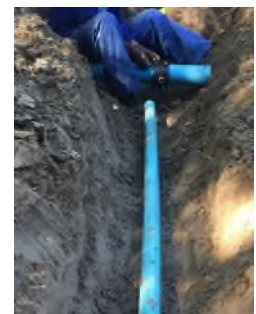
Installing appropriately sized piping with secure connections
